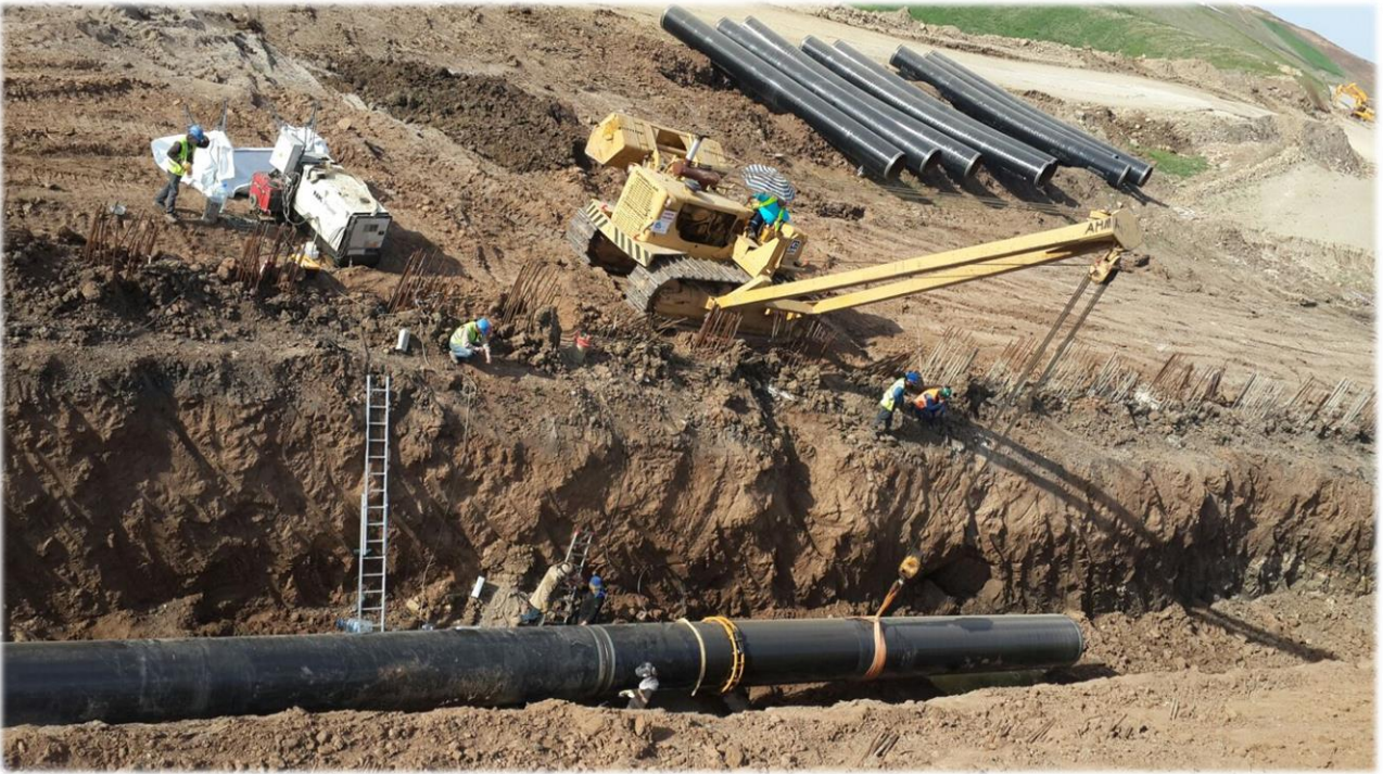
ANKARA-SİVAS DEMİRYOLU PROJESİ 48" MAVİ AKIM DOĞALGAZ BORU HATTI DEPLASMANI RELOCATION OF 48" BLUE STREAM BOTAS NATURAL GAS PIPELINE WITHIN THE SCOPE OF ANKARA-SİVAS RAILWAY PROJECT
