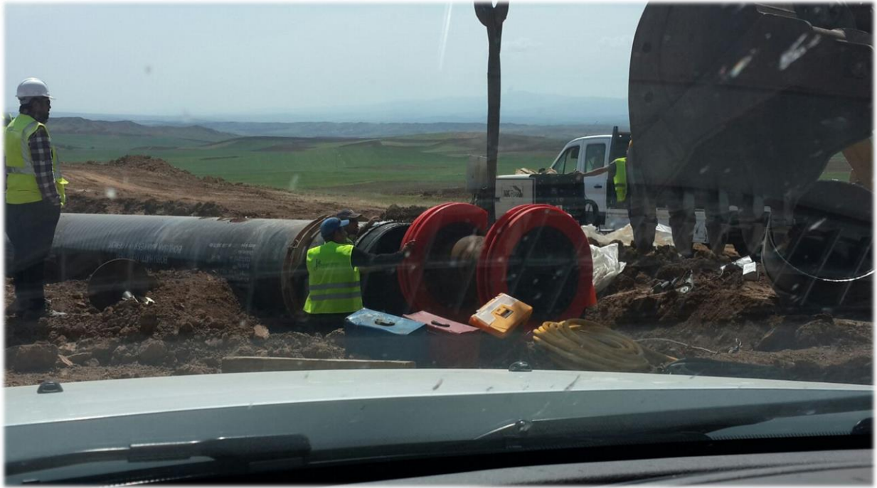
ANKARA-SİVAS DEMİRYOLU PROJESİ 48'' DOĞALGAZ BORU HATTI DEPLASMANI RELOCATION OF 48'' NATURAL BOTAŞ PIPELINE WITHIN THE SCOPE OF ANKARA-SİVAS RAILWAY PROJECT
