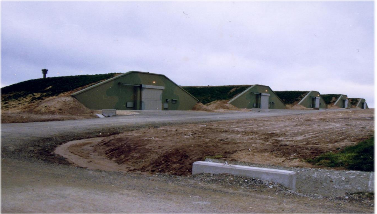
38.DİLİM 1.GRUP İ.D.T.İNŞAATI İŞİ KAPSAMINDA MAYIN DEPOLARI MINE YARDS
