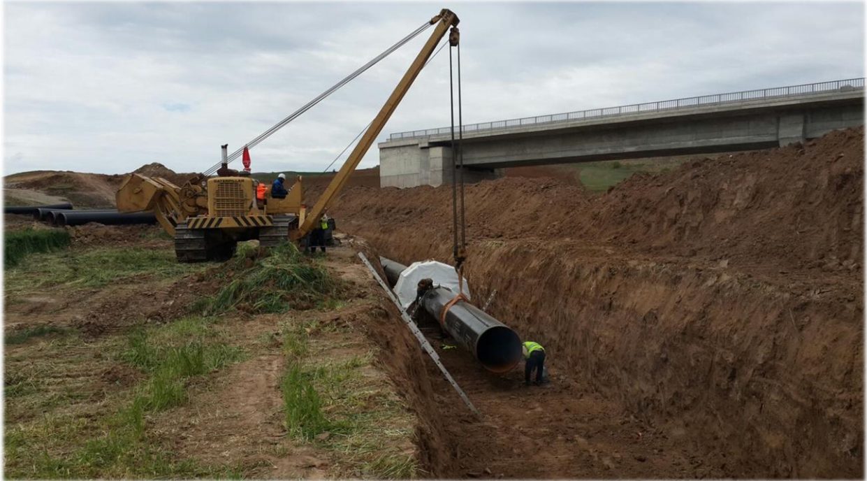
ANKARA-SİVAS DEMİRYOLU PROJESİ 48'' MAVİ AKIM DOĞALGAZ BORU HATTI DEPLASMANI RELOCATION OF 48'' BLUE STREAM BOTAŞ NATURAL GAS PIPELINE WITHIN THE SCOPE OF ANKARA-SİVAS RAILWAY PROJECT
